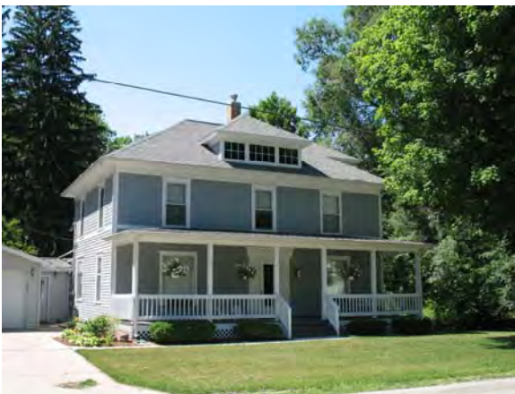
115 Main Street, Whitehall Swedentown Boarding House
