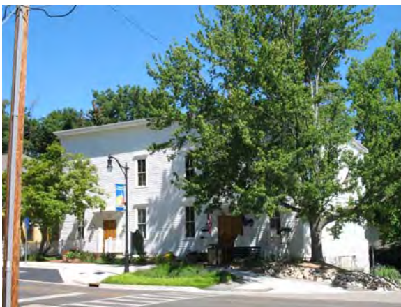
Center Avenue, Douglas Douglas Town Hall
