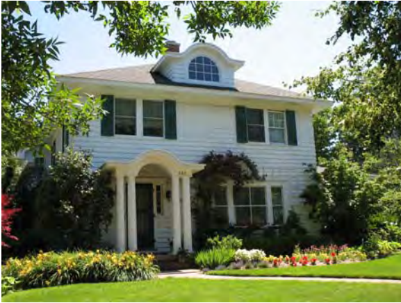
507 Butler Street Residence
